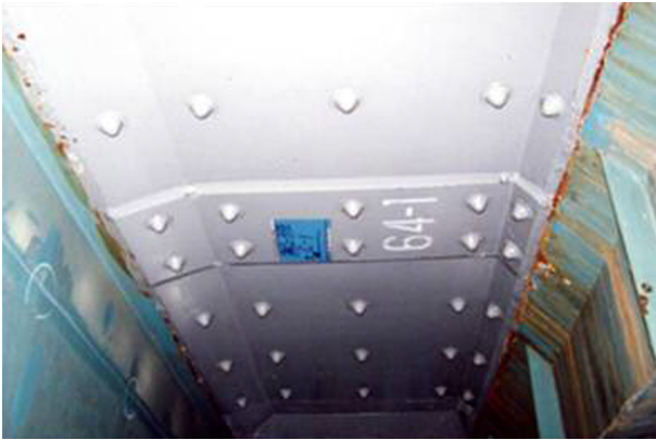
Fig. 1. RC slab bonded with steel-plates.
