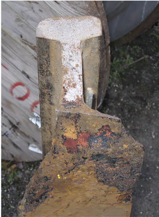
Fig. 1. Corrosion of the rail foot commonly found within level crossings with little or no loss in rail depth.
