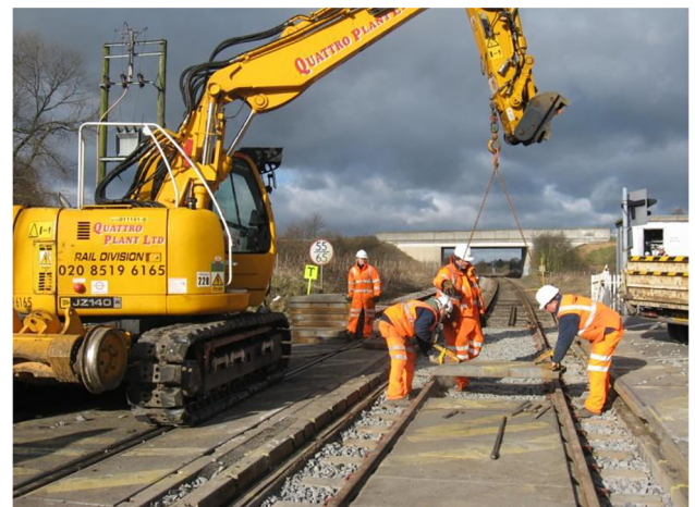
Fig. 3. Lifting the deck to allow visual inspection of the rail.
