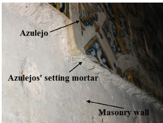
Fig. 2. Azulejos coating system.
