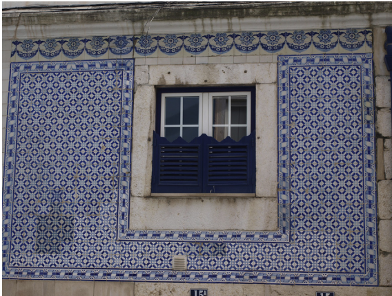
Fig. 1. Azulejos facade coating of a building in Calçada do Cardeal, Lisbon.
