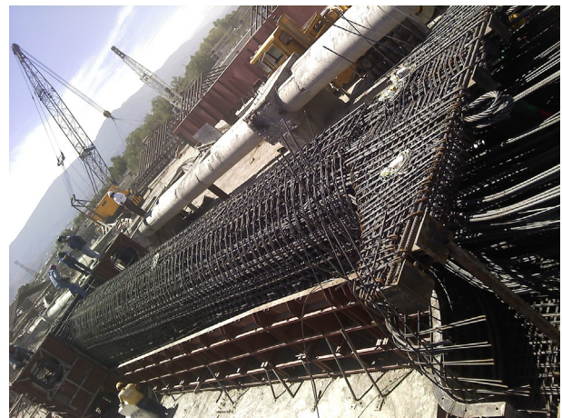
Fig. 1. Monitoring column footing ZC049 during its production.
