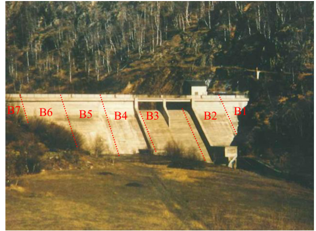
Fig. 1. View of the dam from downstream.
