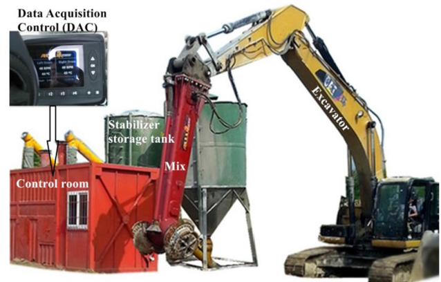
Fig. 1. In-situ mud stabilization system.
