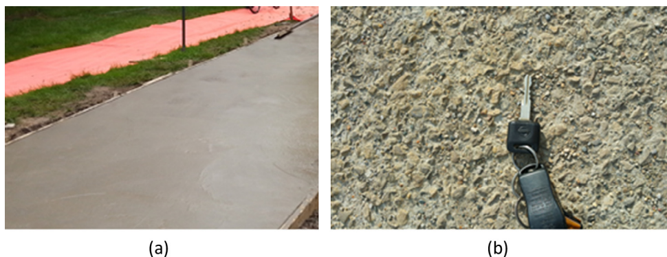
Fig. 1. (a) Picture of the sidewalk cast in summer; and (b) the extensive deicer salt scaling experienced after six months.
