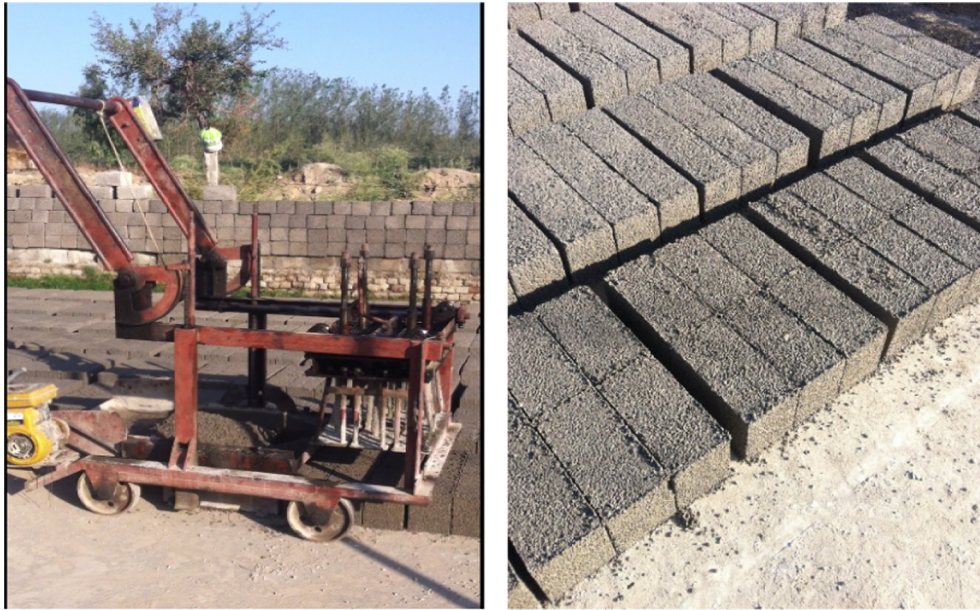
Fig. 1. CMU manufacturing operations in a small scale production facility.
