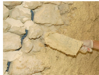
(b) Coating with a trowel ( 800 - 900 \text{ kg}\cdot\text{m}^{-3} ).
