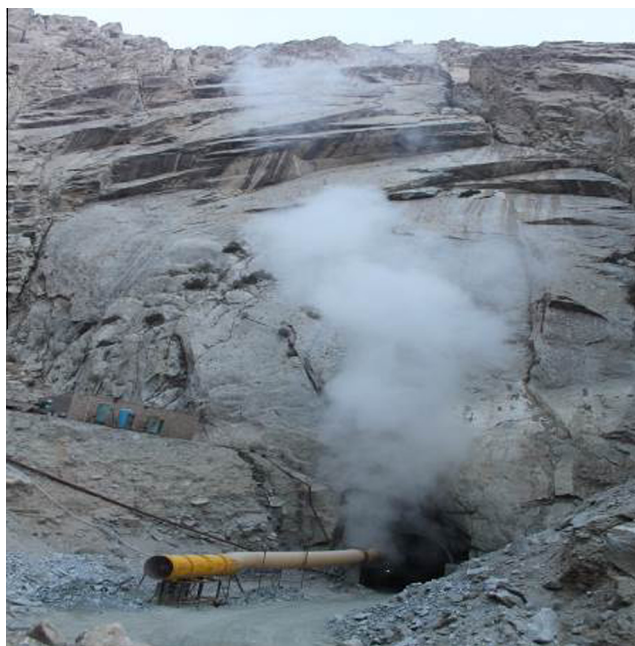
Fig. 1. Water vapour gushing into the entrance.
