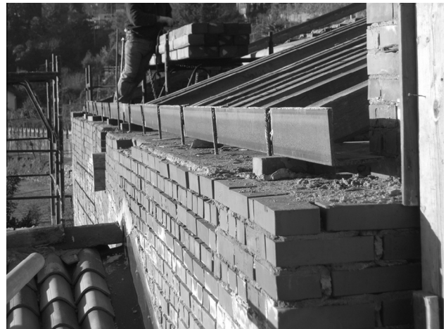
Fig. 4. Example of a steel-profile ring-beam.
