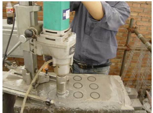
(b) Drilling core sampling
