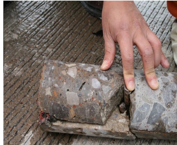
Fig. 1b. Shear failure of tie bar.
