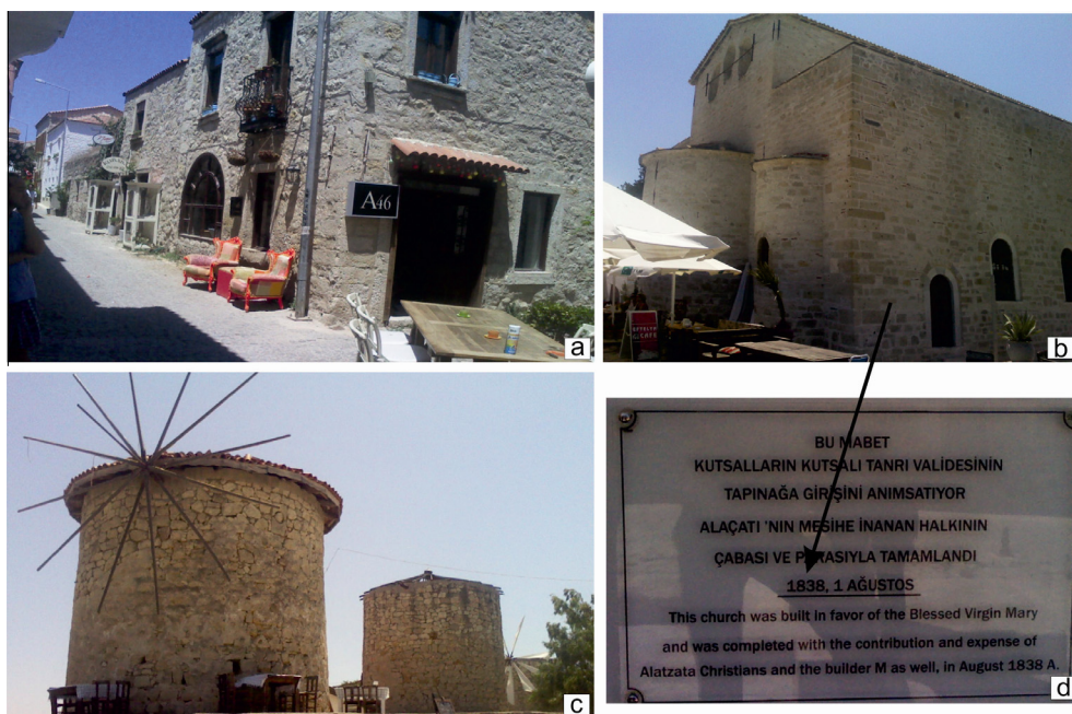
Fig. 1. Examples of historical buildings constructed in Alaçatı with tuff: (a) historical house, (b and d) historical church that was built in 1838; and (c) abandoned historical wind mills.
