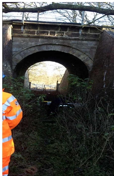
Fig. 3. Whiley Hill bridge.
