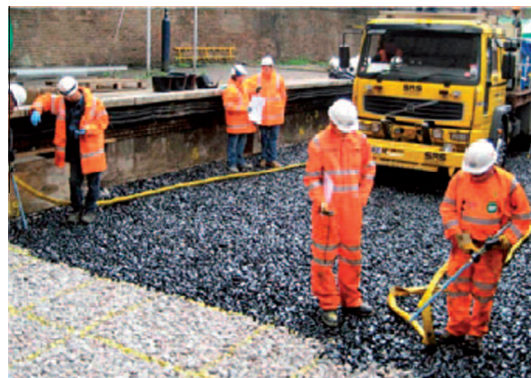
Fig. 1b. Polymer application with the rails removed.
