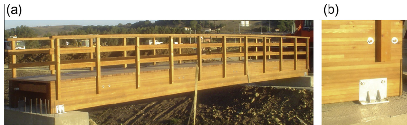
Fig. 1. (a) Picture of a typical timber footbridge in Spain; (b) detail of the steel fastener (support A).
