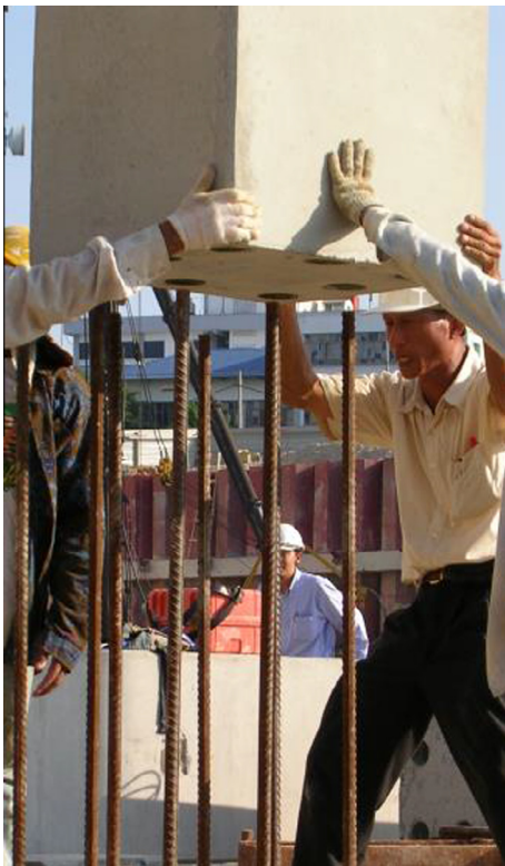
Fig. 2. Grouted sleeve connection.
