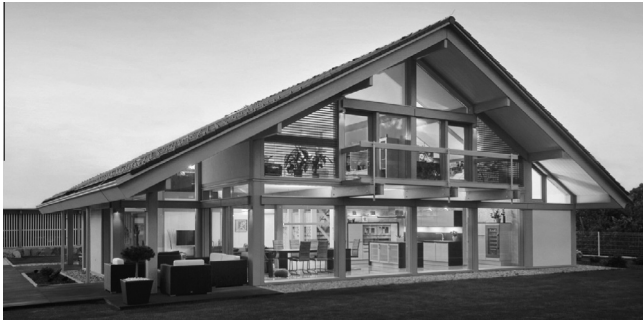
Fig. 1. Timber–glass residential building with a large south-oriented glazing area (photo archive of the company Kager).
