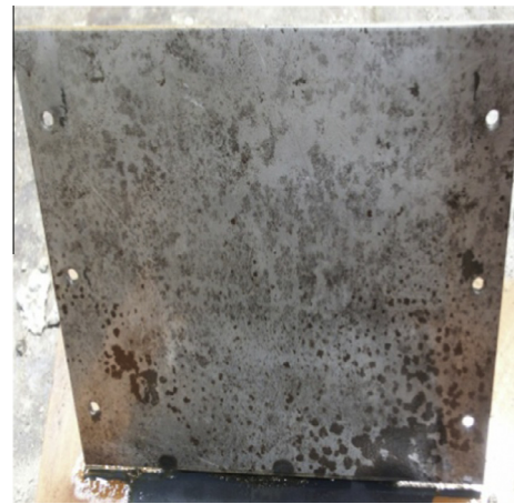
Fig. 3. Used formwork surface.
