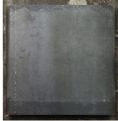
Fig. 2. New formwork surface.
