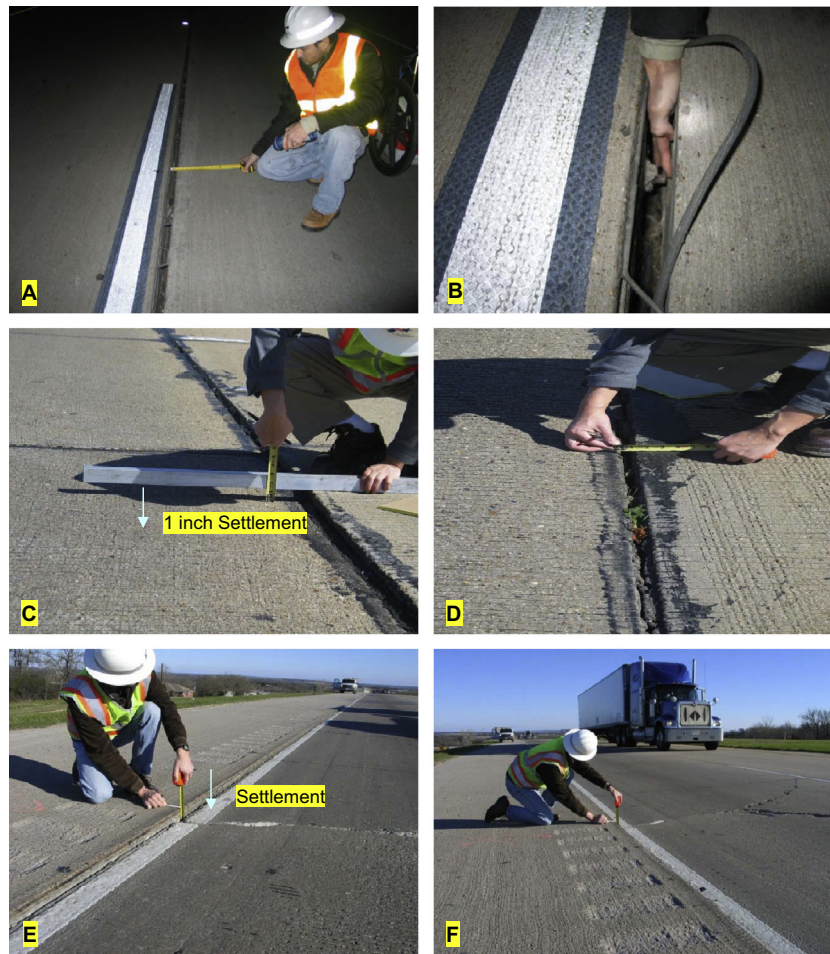
Fig. 1. Typical examples of lane separation, faulted and shattered slabs. (A) and (B) Lane separation for IH35. (C) and (D) Faulted JCP slabs on US59-Atlanta district. (E) and (F) Faulted and shatter JCP slabs on US75-Paris district.
