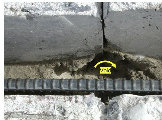
Fig. 3. Void and cracks near the joint.
