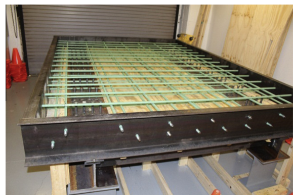
Fig. 2. Deck with rebar and formwork.
