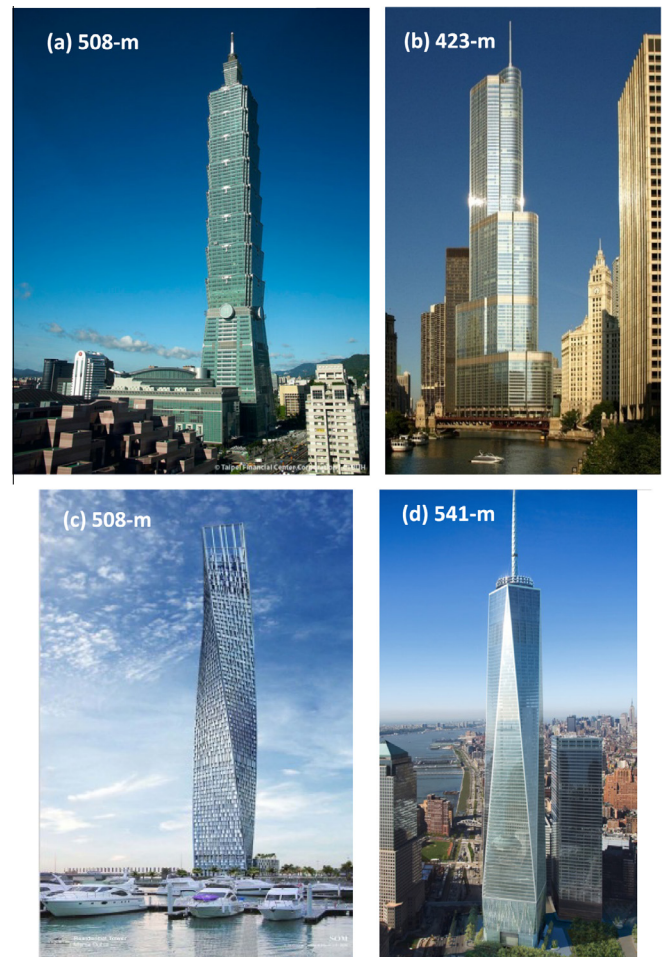
Fig. 1. The (a) Taipei 101 (Taiwan), (b) Trump Tower (Chicago), (c) Infiniti Tower (Dubai), and (d) Tower One, World Trade Centre New York all used SCC in their construction (Photos from [3]).
