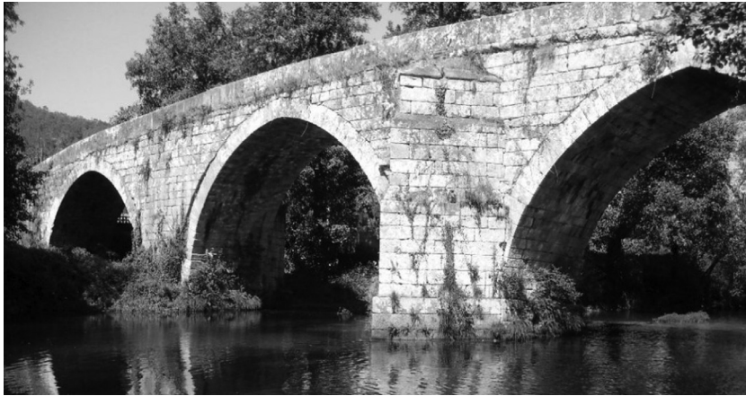
Fig. 1. The Cernadela Bridge.
