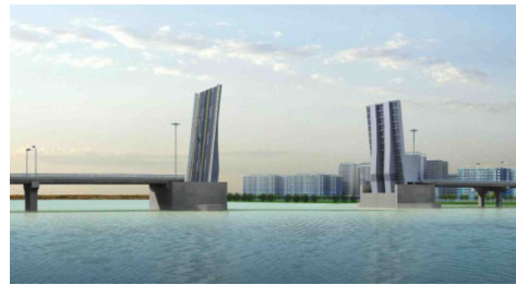
(2) Open state of the bridge
