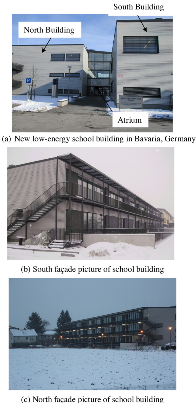
Fig. 1. Façade pictures of low energy building including north and south buildings and atrium (a), south (b) and north (c) sides in winter.
