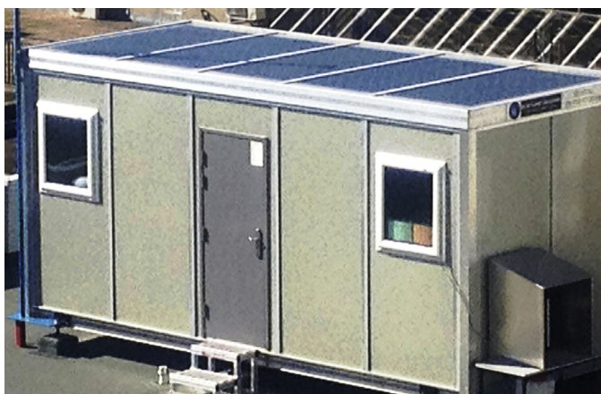
Fig. 1. Solar cabin where PV panels are flat mounted on the rooftop.
