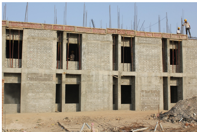
Fig. 1. FaL-G brick masonry building (confined masonry walls).
