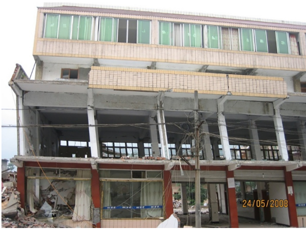
Fig. 1. Weak story failure of RC MRFs in Wenchuan earthquake in China.
