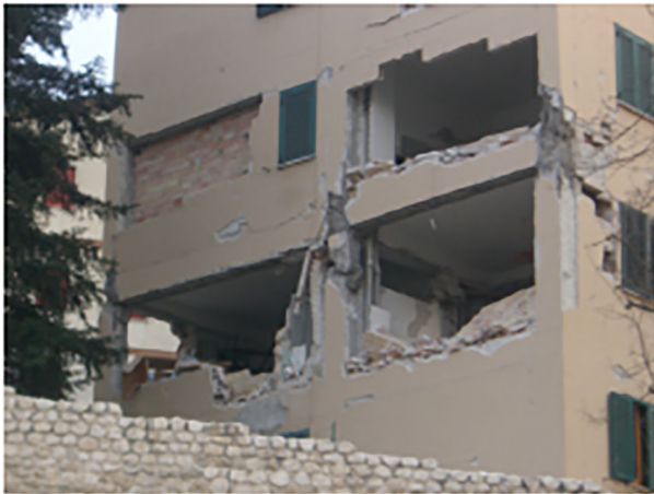
Fig. 2. Out of plane infill wall failure.
