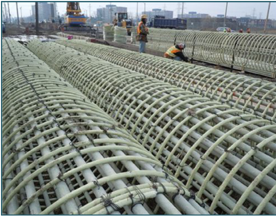
Fig. 1. GFRP cages fabrication and pile soft-eye driving process.
