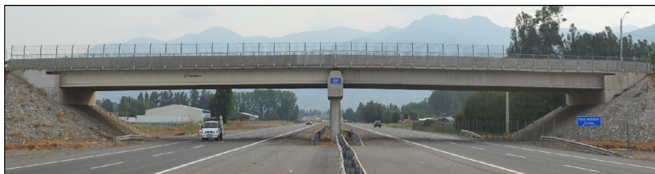
Fig. 2. Case study, Chada underpass (repaired structure after the 2010 Maule earthquake).
