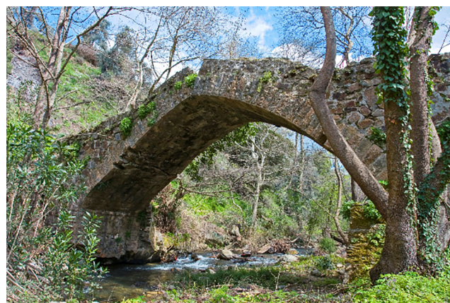
Fig. 1. Kakodiki Bridge: general view from the downstream side [4,5].
