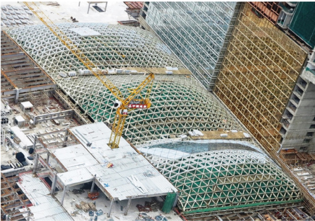
(a) Overall View
