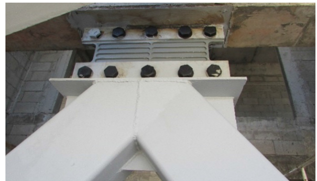
Fig. 2. Installation of a SL for the new construction of Torre Ixtapa (Mexico).
