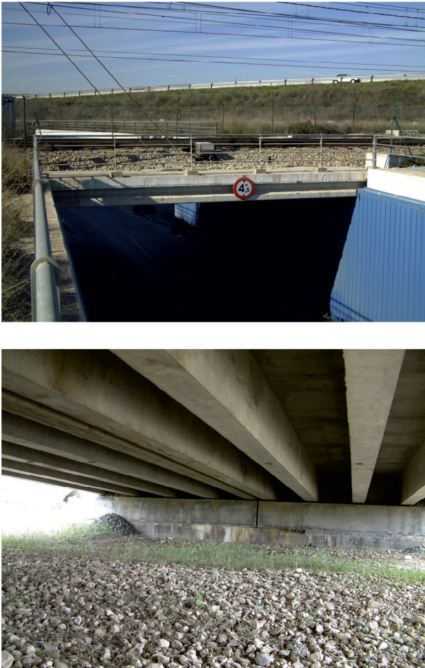
Fig. 1. Railway bridges in Spanish lines composed by simply-supported bays of short-to-medium span.
