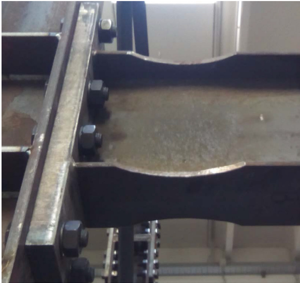
Fig. 1. Typical shape of a “Dog-Bone” connection.
