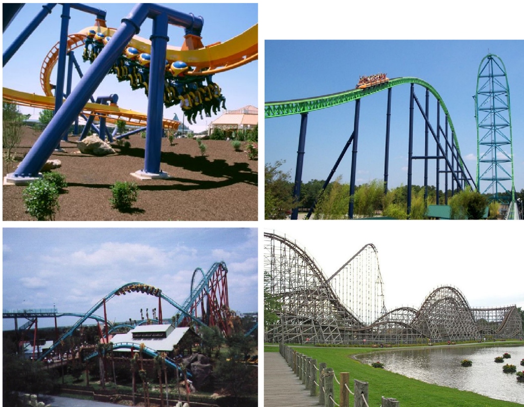
Fig. 2. Example of some roller coaster supporting structures typologies.
