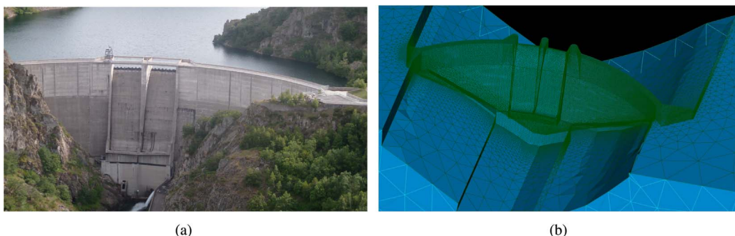
Fig. 1. (a) Photography of the dam and (b) finite element mesh.
