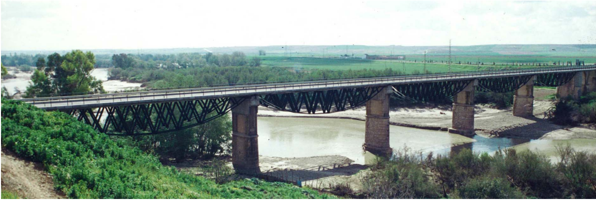
Fig. 1. E. Torroja's bridge in Posadas, Córdoba (Spain).
