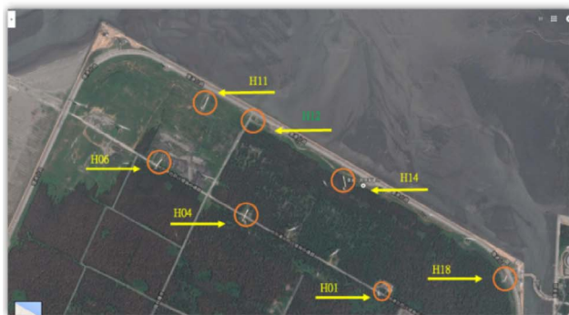
Satellite image (after turbines collapsed)
