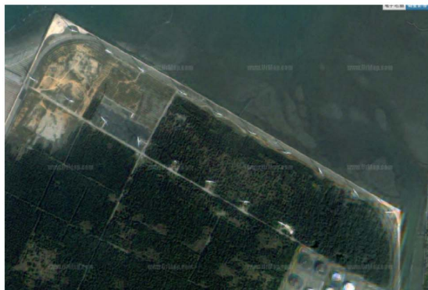
Satellite image (before turbines collapsed)
