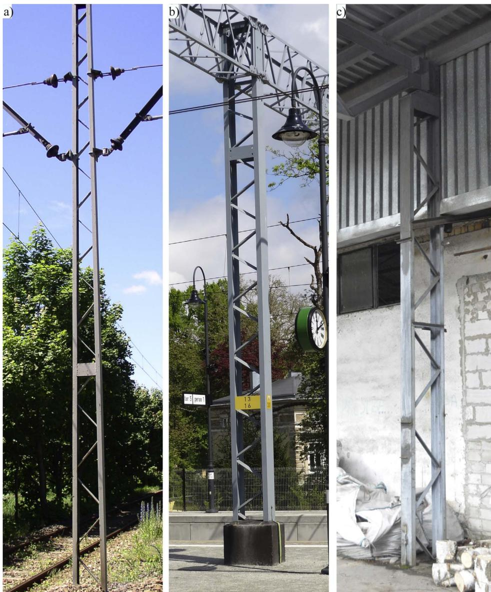
Fig. 1. View of: (a) tramway overhead contact line pole, (b) railway overhead line gantry column, (c) industrial hall column.
