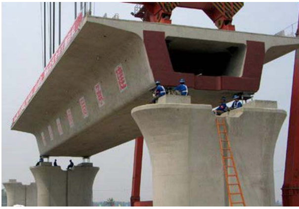
Fig. 1. A thick-walled haunched trapezoidal cross section with wide flange slabs.
