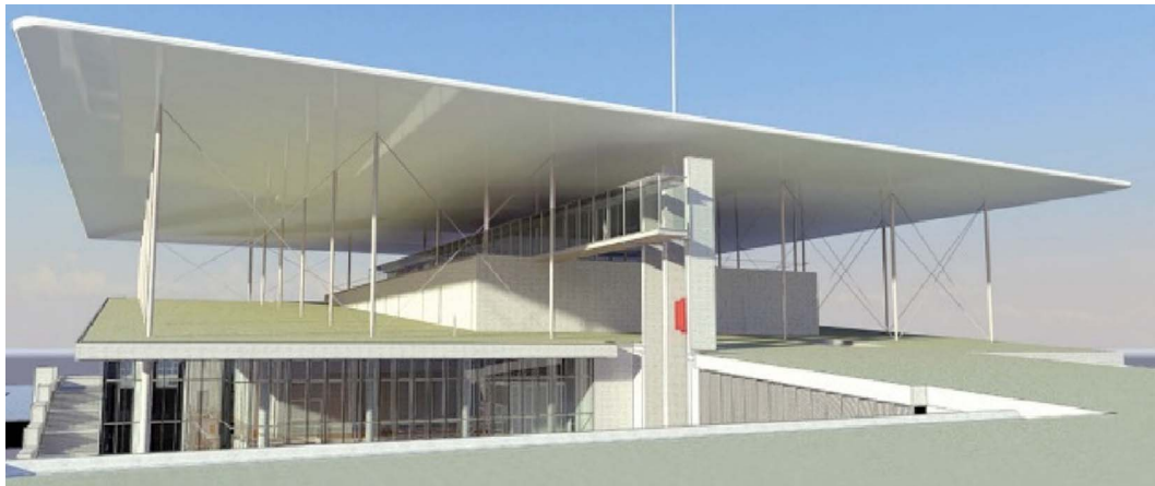
Fig. 1. The SNFCC with the 100 \times 100 ferrocement canopy roof.
