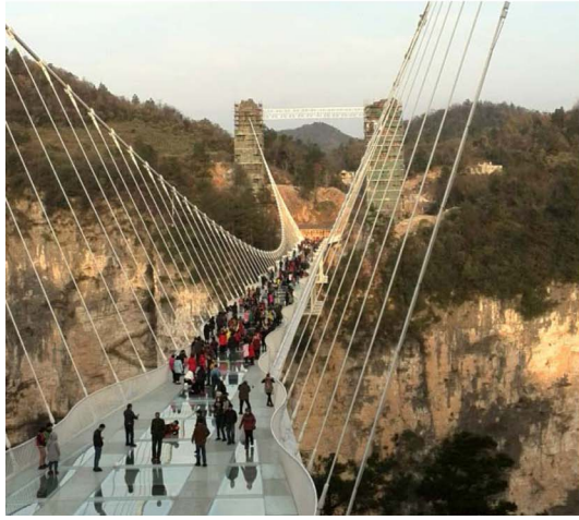
(a) Pedestrian cable-supported bridge
