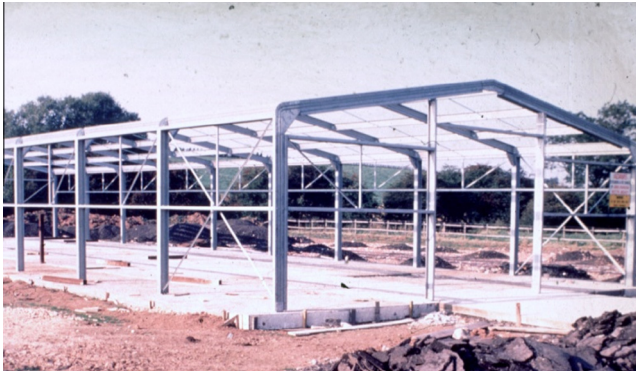
Fig. 1. Typical cold-formed steel portal framing system.
