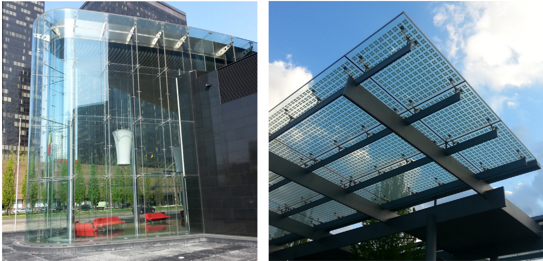
Fig. 1. Federal Public Service Finance in Brussels and bus terminal in Kaiserslautern.
