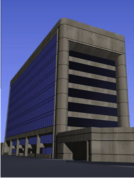
Fig. 1. North view of MFB before collapse (courtesy: John D. Osteraas).
