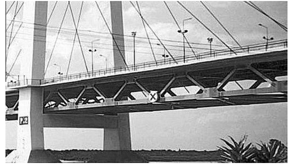
Fig. 2. Trussed deck of cable-stayed bridge.
