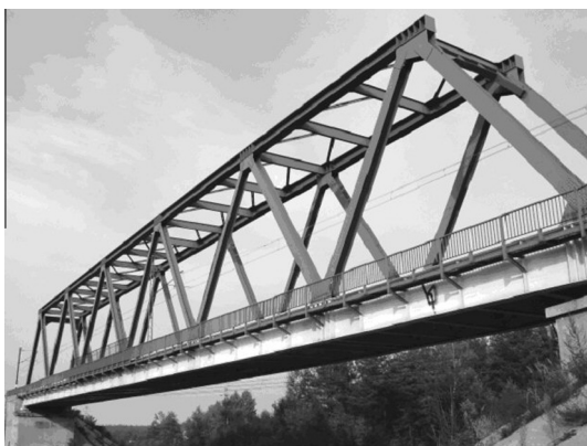
Fig. 1. Trusses as main girders.
