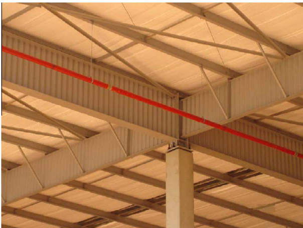
Fig. 1. Roof supported by sinusoidal-web girders.
