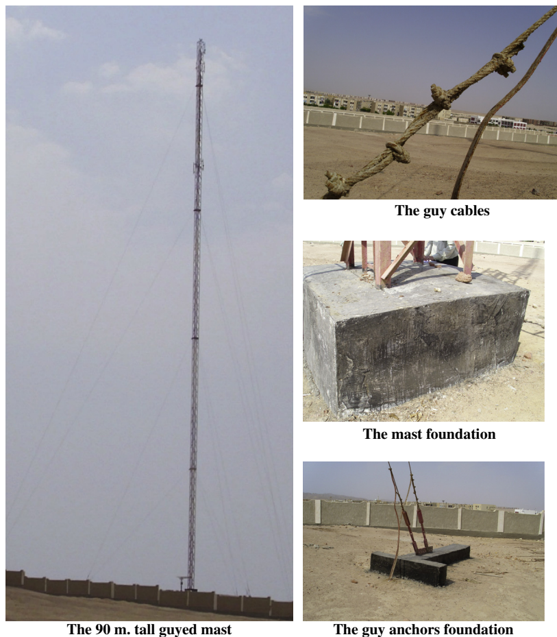
Fig. 1. The components of the guyed mast.
